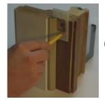
Install the Template using the Striker-plate screws and mark the inside of the rectangular hole. Then remove Template.
