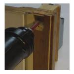
Remove the marked area, including the pencil mark. This may be done by wood chiseling, using a hand router, etc. Route the hole 1 ½" deep.
