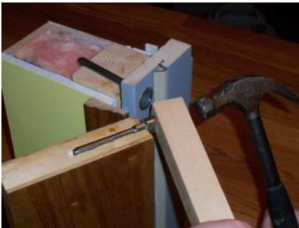
11 Apply appropriate glue to Detail #2 and install into edge of door making sure the radius of the "Head" is in line with the swing arc of the door as it closes. Seat Detail #2 with a block of wood and hammer.
