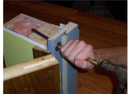
10 There is a designed interference in the last 1/4" of Detail #1. Seat Detail #1 in position with a punch and hammer.
