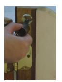
Apply an appropriate glue to the smaller diameter of the female socket. Insert it into the hole, rotating to align the larger diameter with the bored hole and the extension with the ½" drilled hole.
