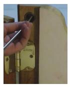
Seat the last ¼" with a punch until the face is flush with the doorframe. Don't drive it in too far, as you will lose effective interlocking with the male pin that will be in the door. Then secure with one of the stainless steel screws supplied with the system.
