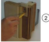
Install the Template using the Striker-plate screws and mark the inside of the rectangular hole. Then remove Template.
