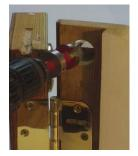
At this punch mark, maintaining horizontal level and perpendicular to the doorframe, Bore a 1 1/8" Diameter hole, 1 ½" Deep.
