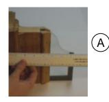
NOTE: Make certain your door has adequate wood structure and proper alignment holding your doorframe to accept our Product. Measure the distance between the door jamb and the framework that holds the sidelight window. There must be at least 2 ¾" to install our product. In this demonstration model we show over 3 ½". (If your door does not have the minimum 2 ¾", you can cut off an appropriate length of the ½" diameter pin extension and adjust your drilling dimensions according.)
