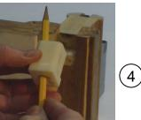
Align the drill guide so the hole will guide the drill toward the exterior of the building as we determined in section "B".
