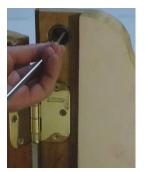
Seat the last ¼" with a punch until the face is flush with the doorframe. Don't drive it in too far, as you will lose effective interlocking with the male pin that will be in the door. Then secure with one of the stainless steel screws supplied with the system.
