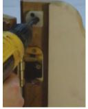
Use a ½" Drill. Keeping the drill level and in line with the Drill Guide angle, drill the ½" hole to a depth of 2 7/8" from the face of the drill guide. You will be drilling at the proper angle to match the angle on Detail #3. Make sure you don't drill too deep to avoid breaking into the glass frame of the sidelight. Then remove Drill Guide
