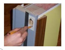
Mark inside the rectangular hole and remove the Template.
