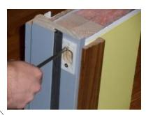
2 Install Template "C" using Striker-plate screws.
