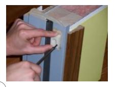
Install Drill Guide "D" and secure with wood screw furnished in kit.
