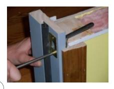
Re-install Striker-plate to cover Detail #3.
