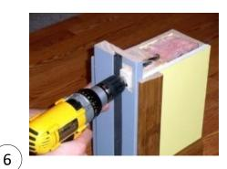
Use a ½" Drill. Keeping the drill level and in line with the Drill Guide angle, drill the ½" hole to a depth of 5 ¼" from the face of the drill guide. You will be drilling at the proper angle to match the angle on Detail #3.
