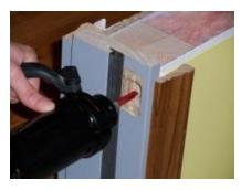
Route the marked area, removing the pencil mark. This may be done by drilling, wood chiseling, or using a hand router. Route or chisel to 1 ½" Deep.
